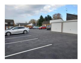
Between 2021 and 2023 the Council has spent around £2m to refurbish garage sites that are to be retained. Works have included demolition of existing garages, resurfacing the hardstanding areas and provision of new larger garages that can accommodate modern vehicles.
